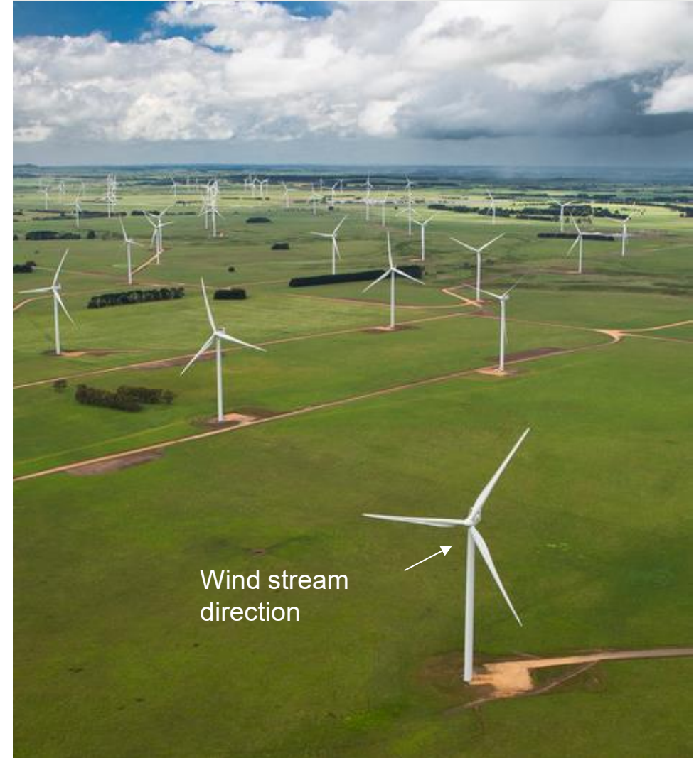
Macarthur Wind Farm, Australia
